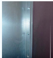
5/16" bolts with serrated lock nut
