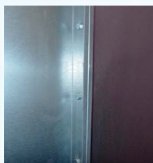
5/16" bolts with serrated lock nut
