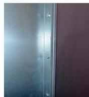
5/16" bolts with serrated lock nut
